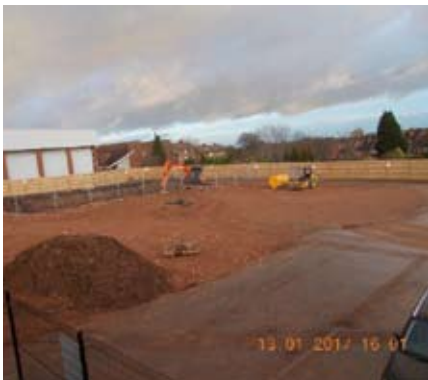
View of cleared site
